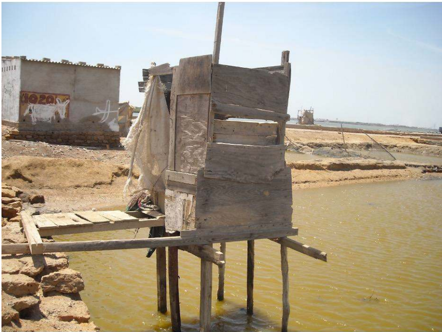
Figure 12: A typical toilet in Rehri Goth
