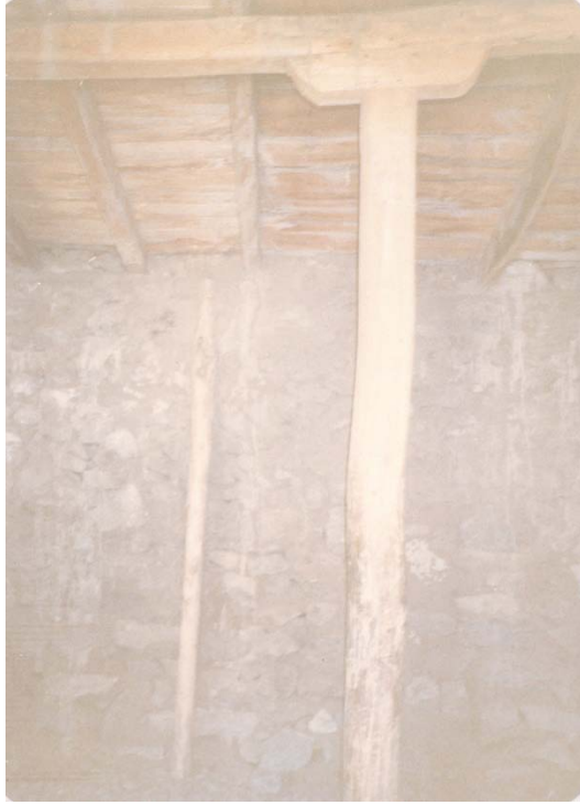
Supports built into the walls : School at Grunjar
