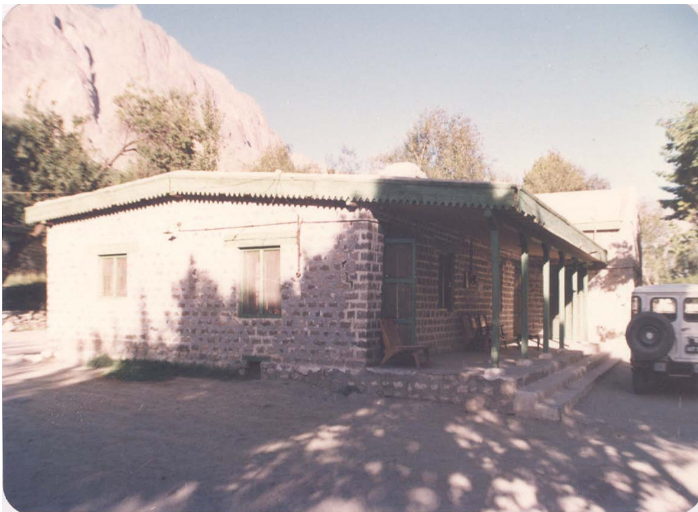
Stone in lime mortar : Gupis Rest House
