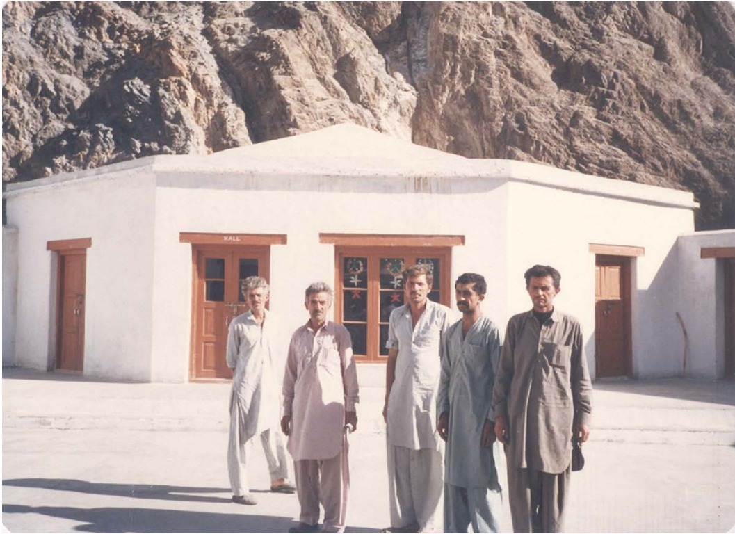
External lime plaster : the school at Khyber
