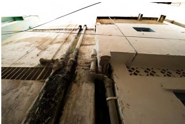
Picture 18: Poor condition of sewerage pipes
