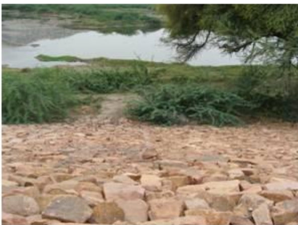
Stone Pitching for Spillway
