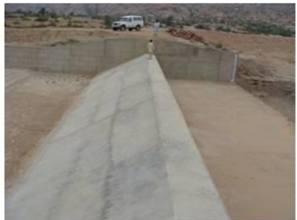
Under Construction SPILLWAY
