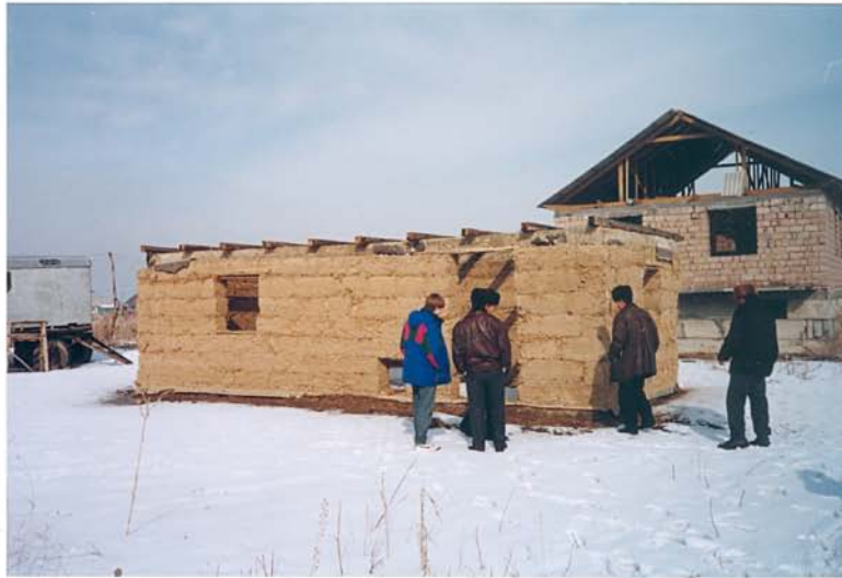
RAMMED EARTH WALL IN LUCHVASTOKA SETTLEMENT
