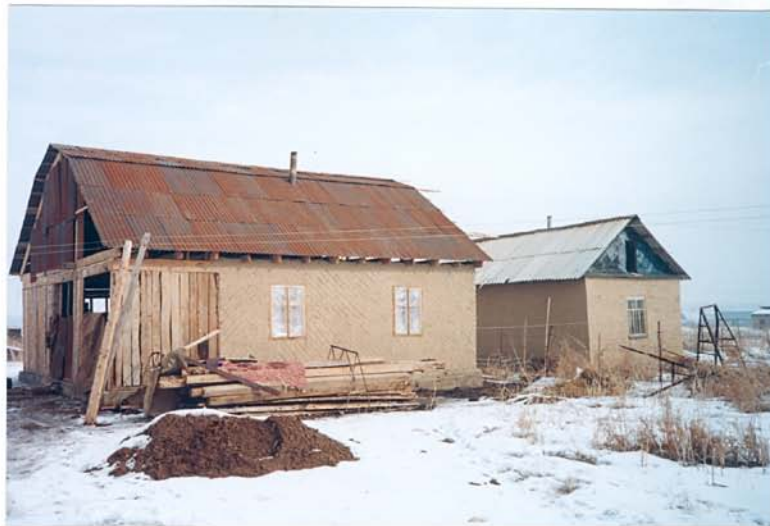
TIMBER HOUSES WITH MUD STRAW PLASTER, LUCHVASTOKA SETTLEMENT
