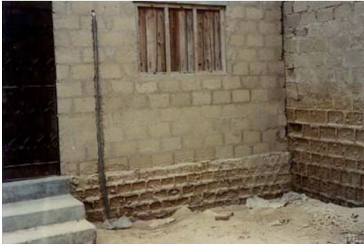
33. Defects in the thalla built housing in Orangi
