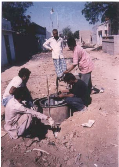
9. Manholes being cast.
