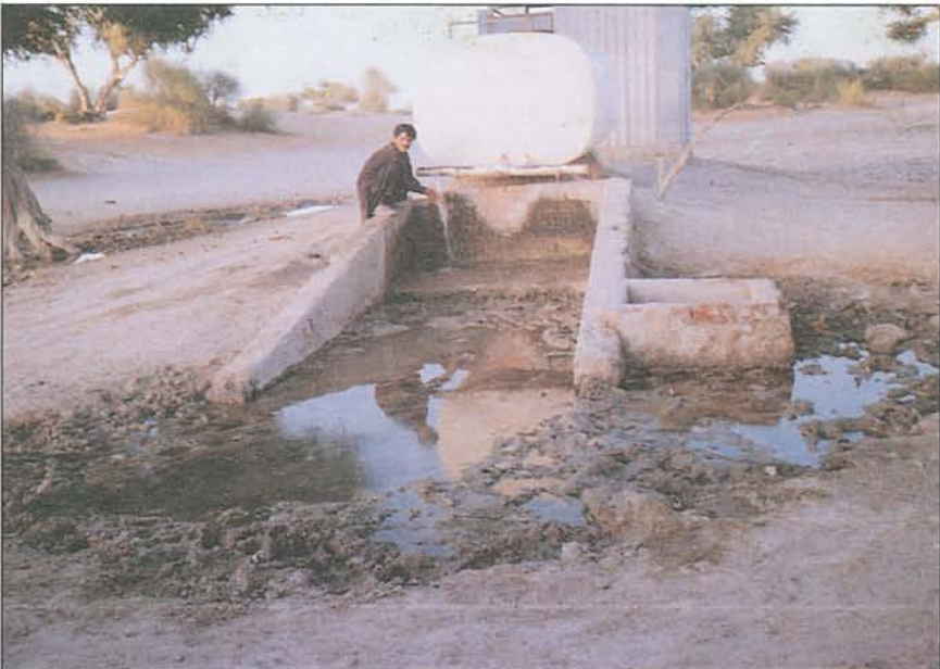
SAZDA water tank in Tarai at Bapuhar
