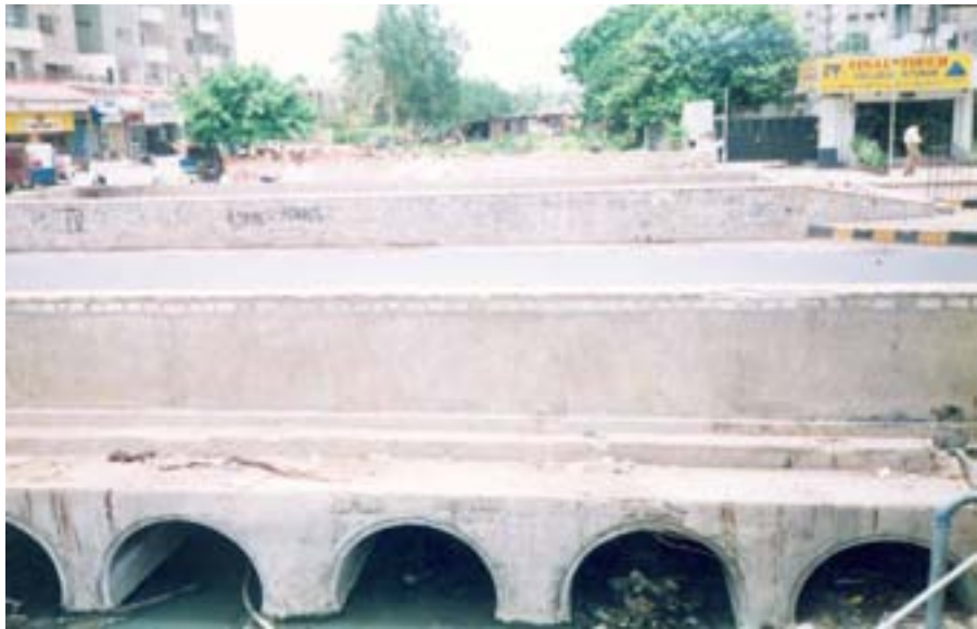
Piped culverts are bottlenecks causing choking - need box culverts
