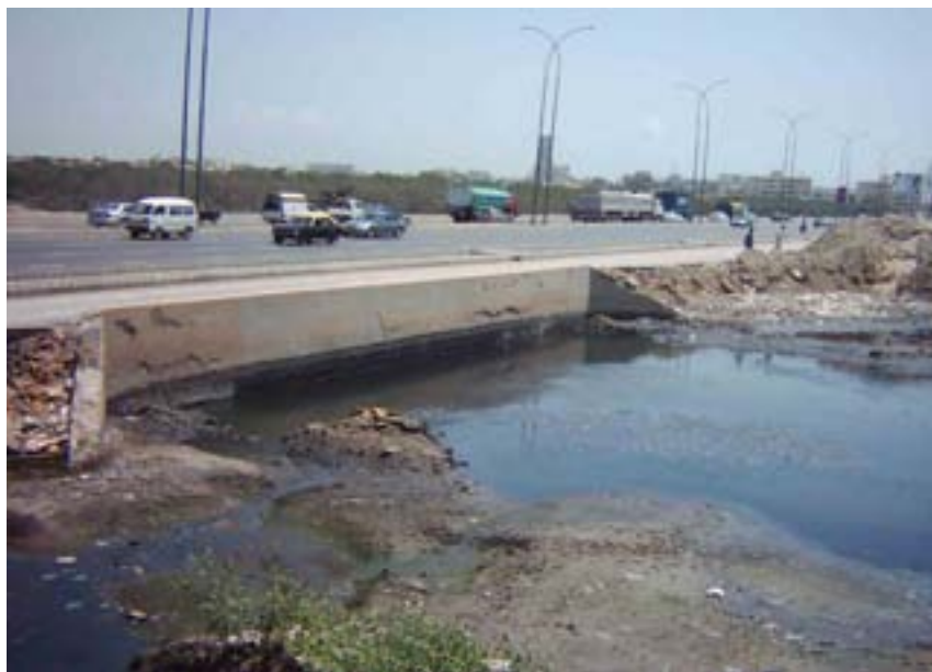
Out fall culvert already choked
