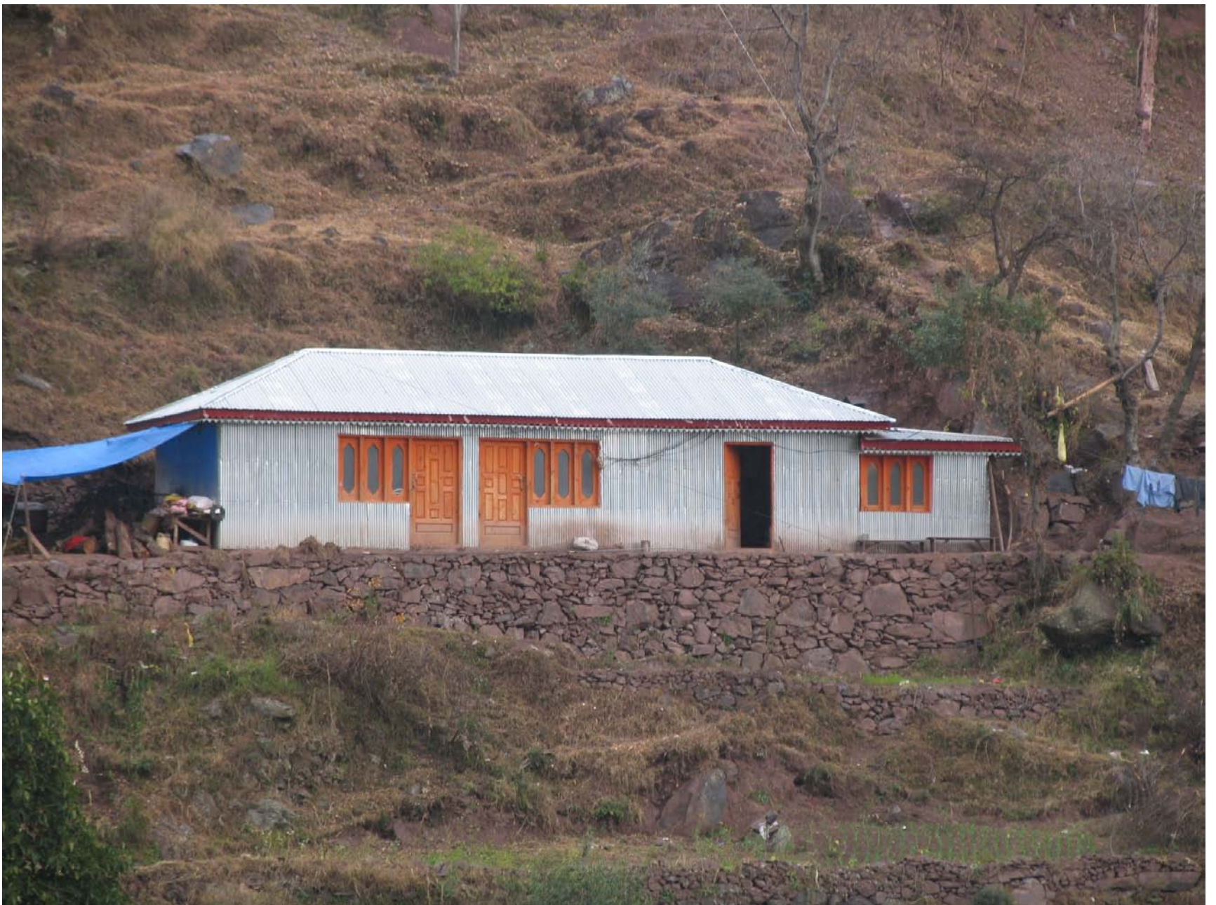
Post-earthquake construction: GI sheet house
