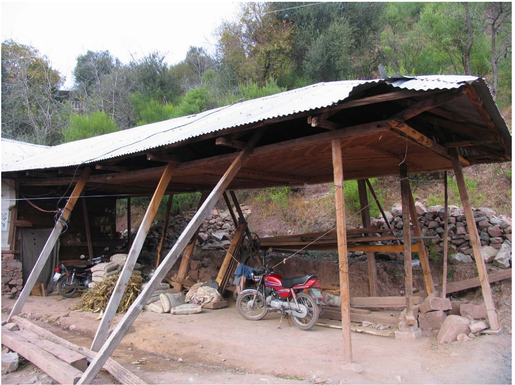
House – 2: The walls collapsed but the roof remained partially intact
