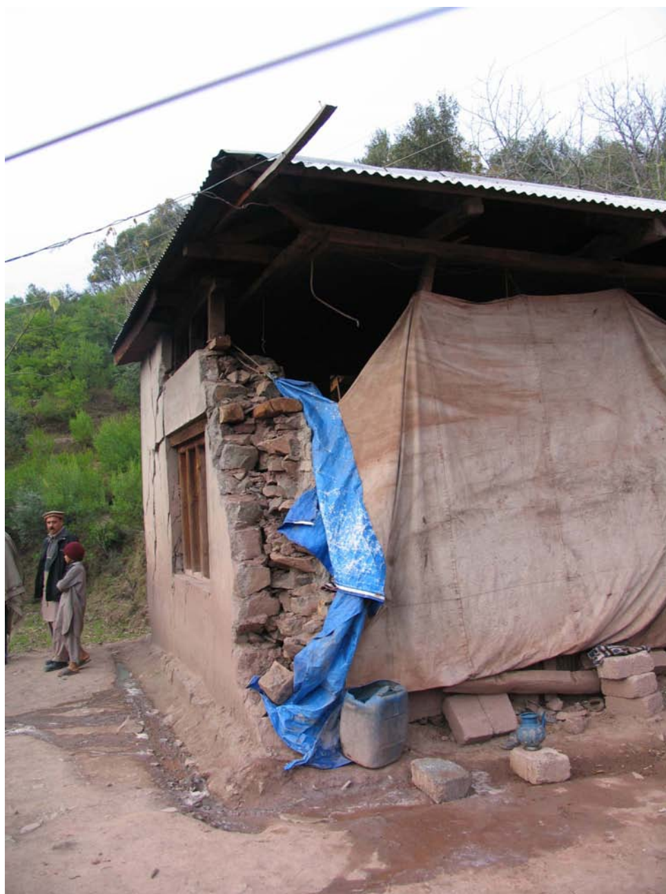
House – 2: Wall construction of the only surviving room
