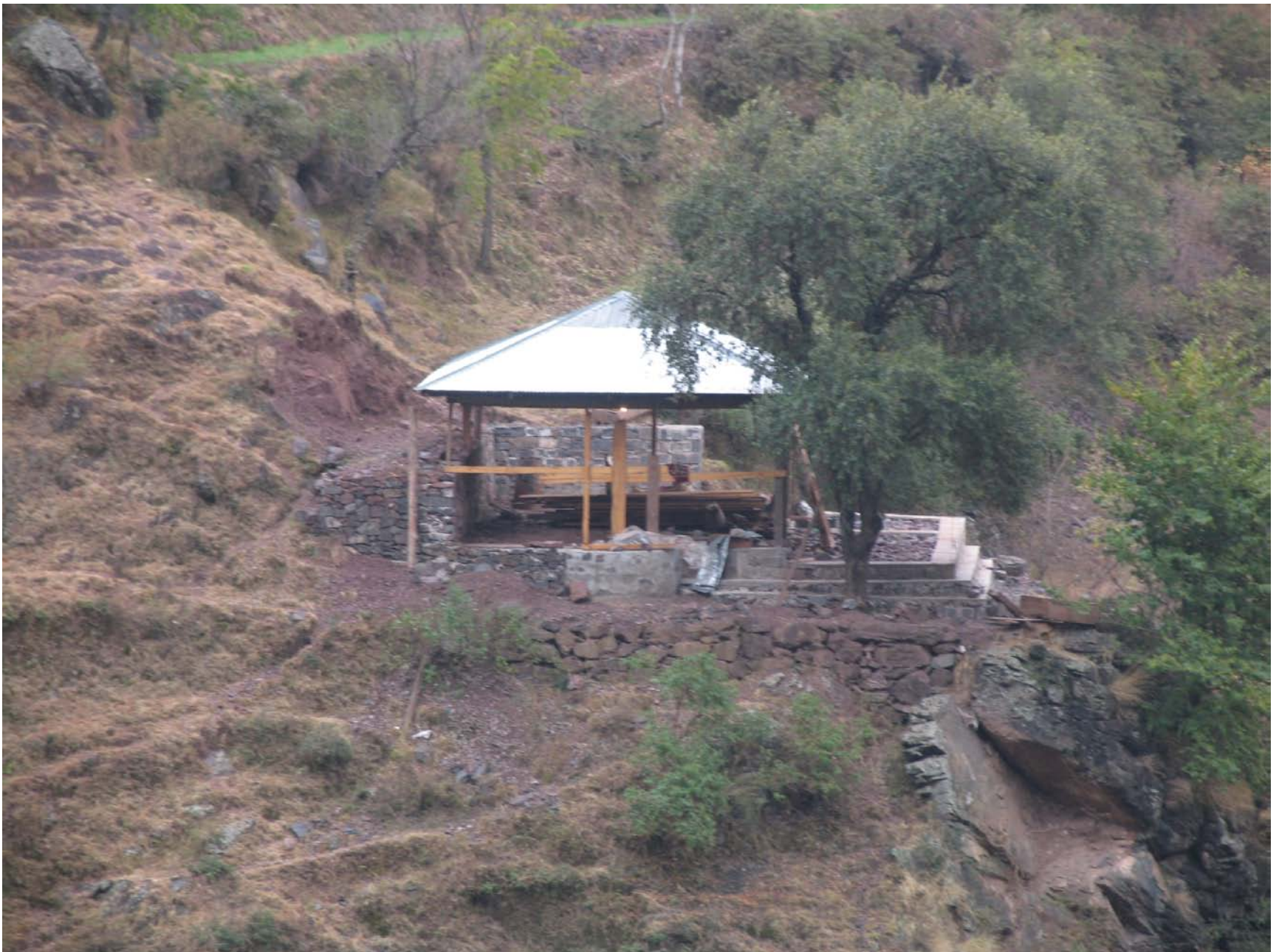
Typical post-earthquake house construction: timber frame, tin roof with concrete block and/or GI sheet walls
