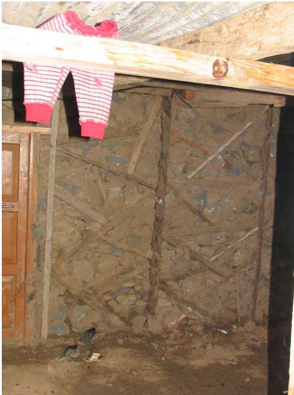
Recently post-earthquake Dhajji construction
