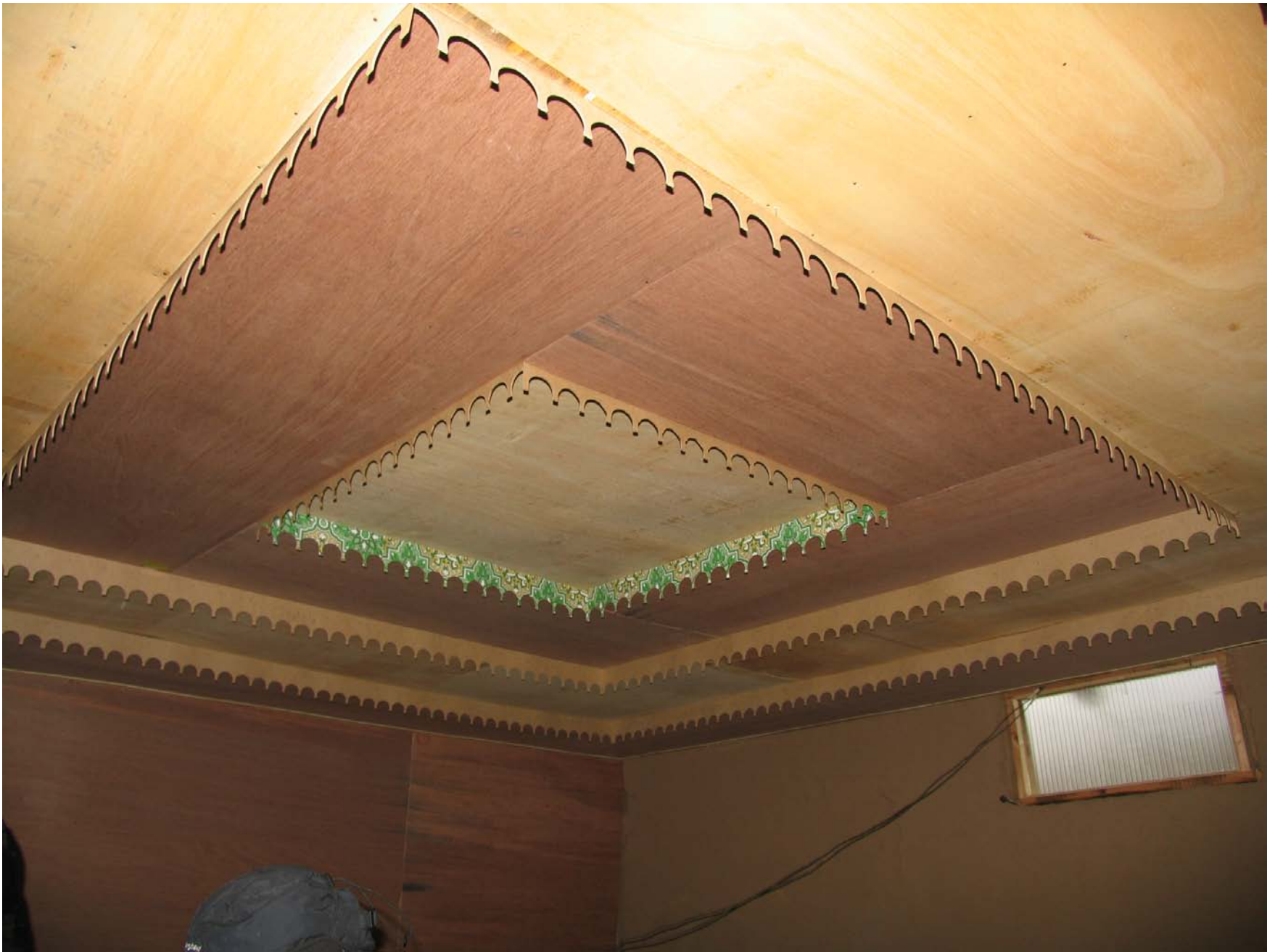
House – 5: False ceiling in plywood
