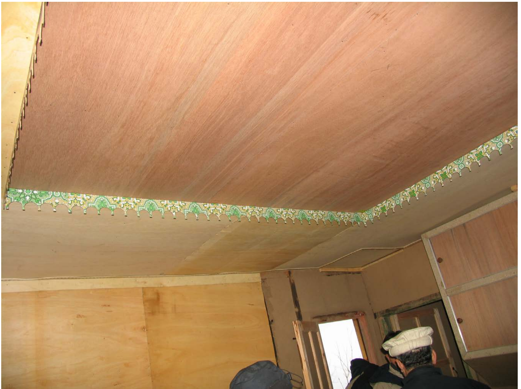
House – 5: False ceiling in plywood
