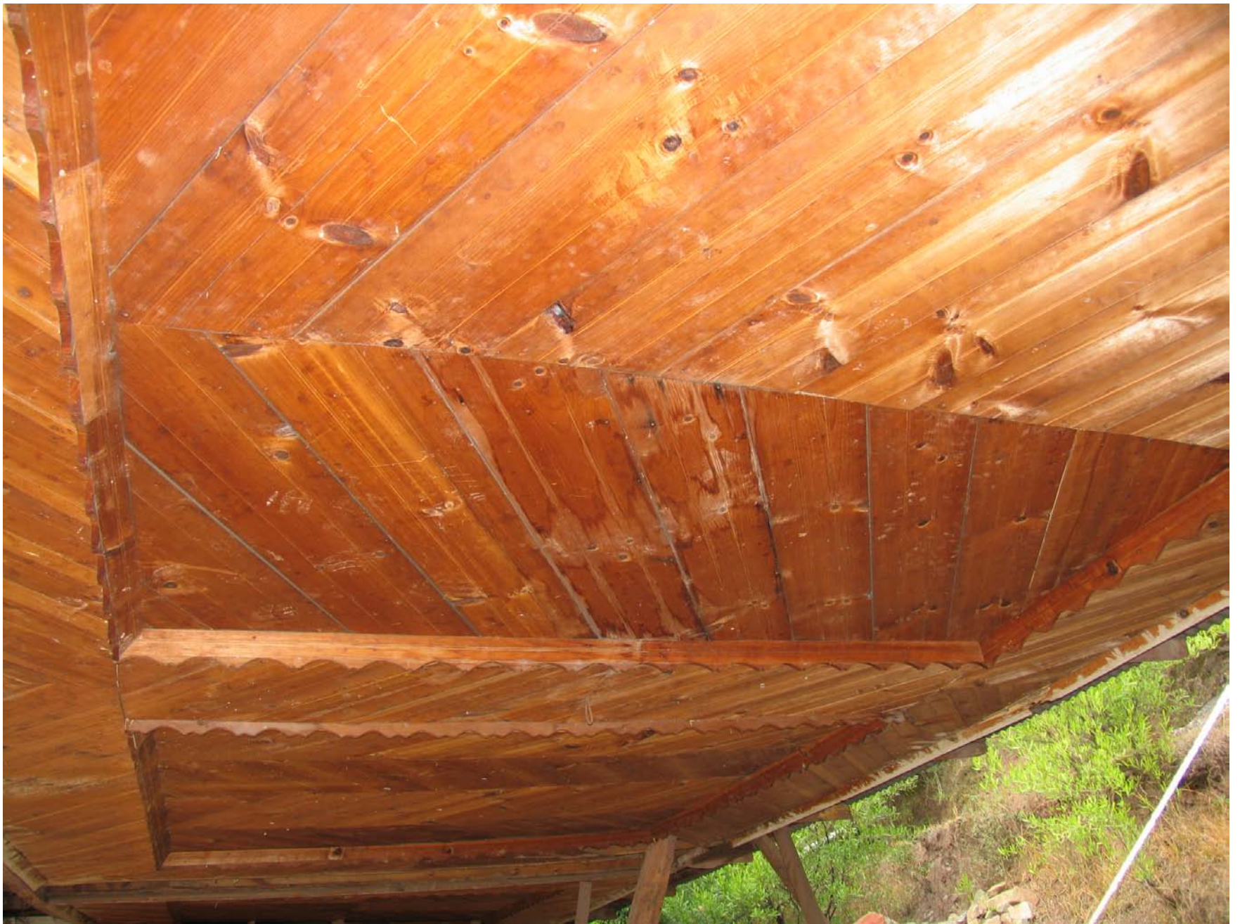
House – 2: Ceiling of the collapsed portion of the house
