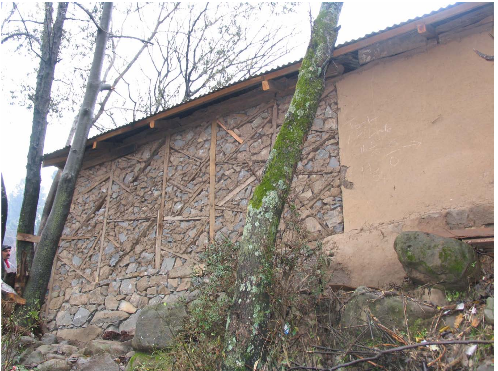
Recently post-earthquake Dhajji construction
