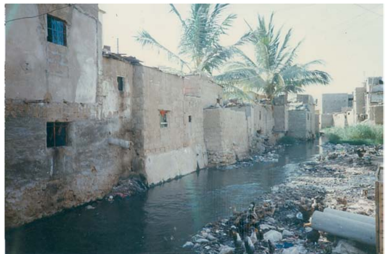
B5-SEWAGE DISPOSAL INTO A NATURAL STORM DRAIN
