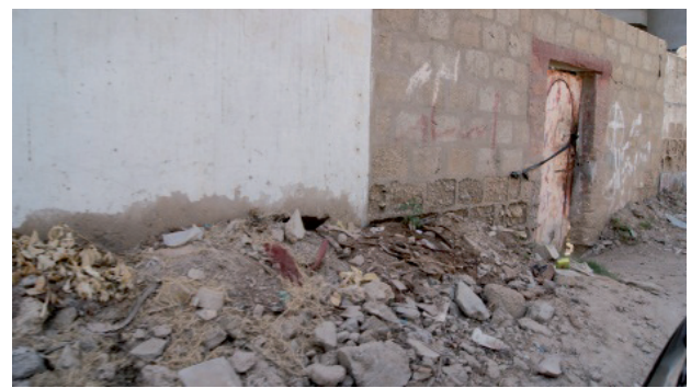
Figure 7. Barrier wall surrounding residence
