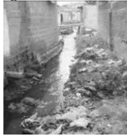
Figure 8: Nalas /drainage channels: a means of sewage disposal
