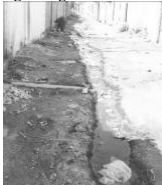
Figure 7: Overflowing sewage in a lane of a squatter settlement
