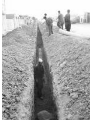
Figure 26: OPP-RTI staff supervising an ADB funded main sewer
