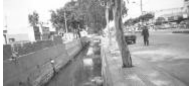
Figure 27: Existing sewerage and drainage system of Korangi
