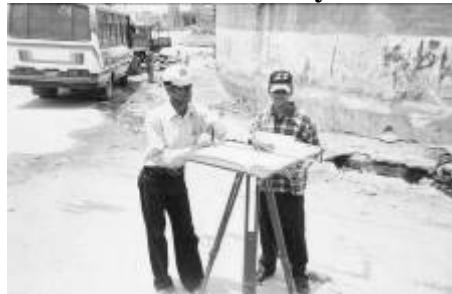
Figure 18: Plane-table survey of a settlement
