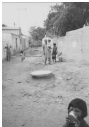
Figure 12: A self-financed lane sewer in Orangi
