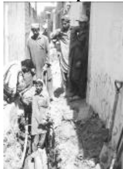
Figure 13: OPP-RTI’s technician providing training support
