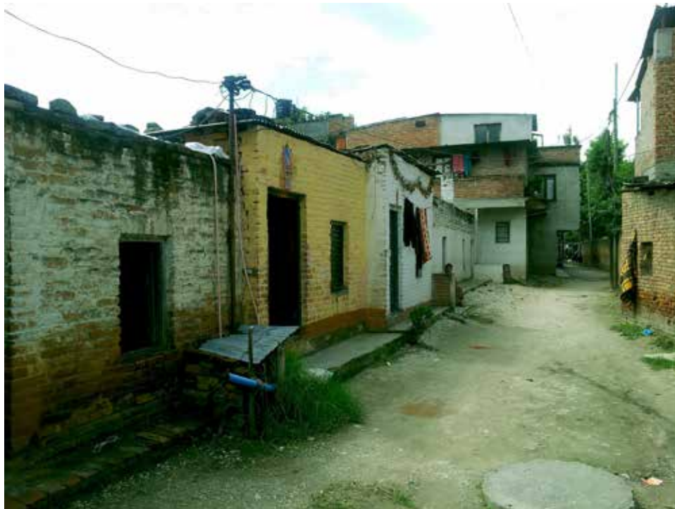
Figure 7. Concrete structures in Sankhamul
